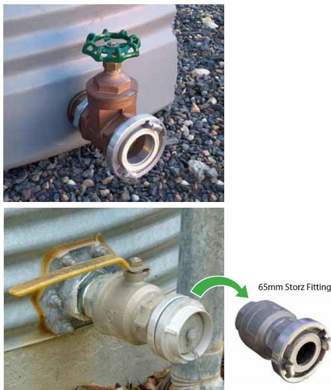
Example of a Storz Outlet with a Gate Valve & a Ball Valve
